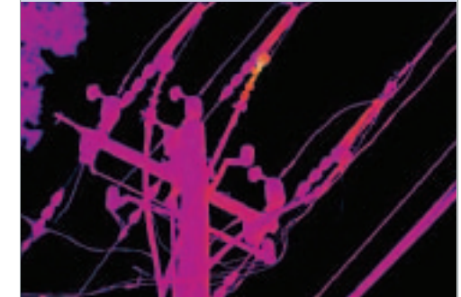
Inspect electrical systems
