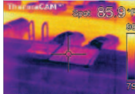
Inspect roofing for leaks and damage
